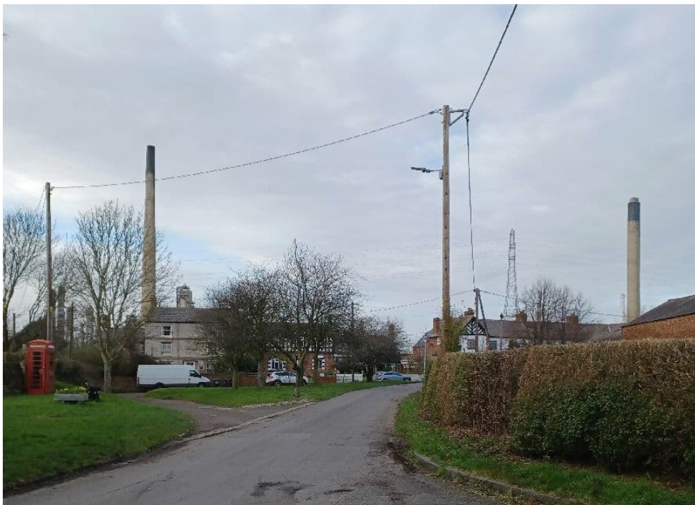
Insert 8.2 - Looking north at Grade II listed Church Farmhouse (NHLE 1330241) within the Thornton-le-Moors CA
